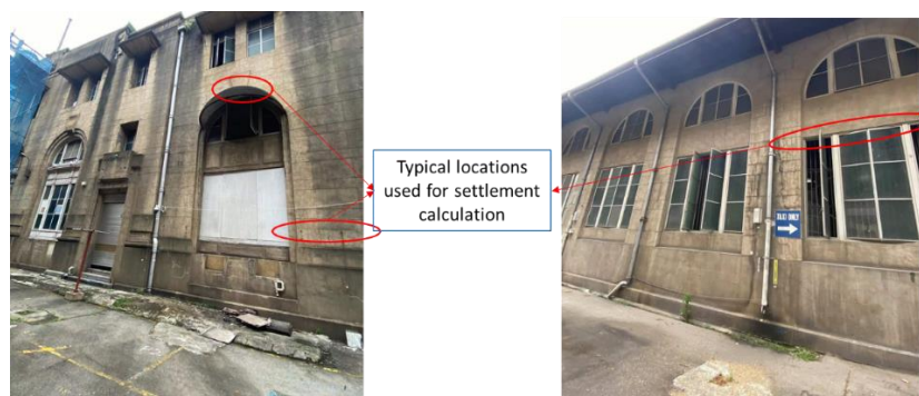
Figure 14. Point selection for building settlement value calculation.
