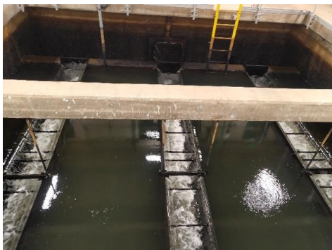
(c) Filter-to-waste backwash
