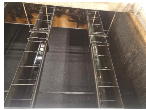
(d) The surface of the water filter medium after backwash
