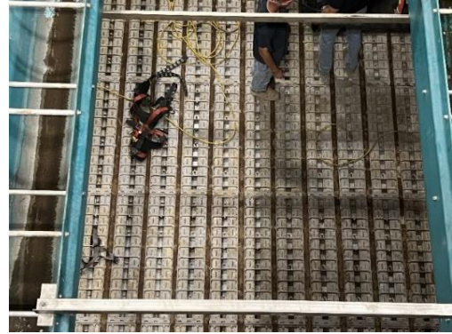
(a) Underdrains inspection
