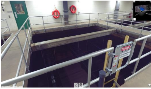
(a) Top of the water filter
