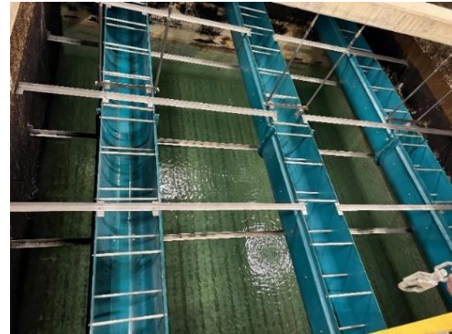
(c) Backwash of underdrain
