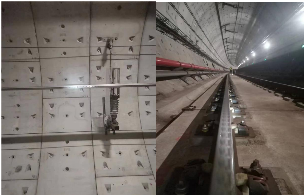
Figure 3. Wave film of contact line between Guangzhou Metro Line 2 and Zhengzhou Metro Line 1.
